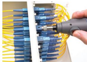
Figure 3-2. Patch panel inspection
