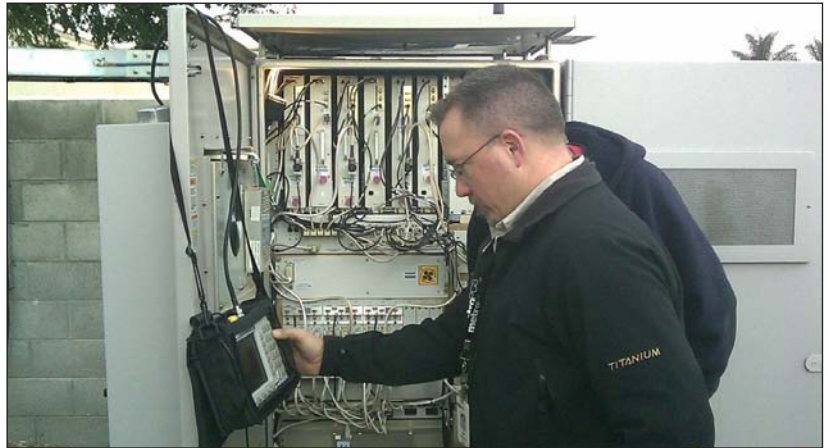
Figure 17: Monitoring a test port on a base station lets you see what the base station receiver is seeing.
